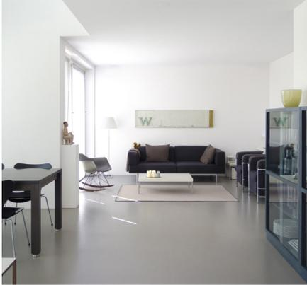
**Synthetic resin floor finishes conduct heat well, making them ideal for use with underfloor heating. They provide a hardwearing, clean, seamless finish, available in a range of colours to suit individual project requirements.**
