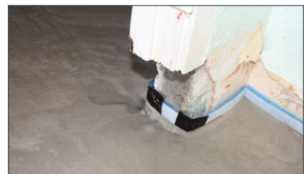
Example of poorly sealed area – self-levelling compound has sunk.
