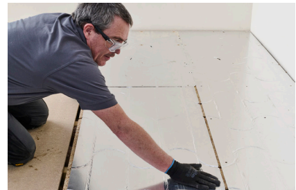
19. Continue to install the boards as shown until the next row is complete.
