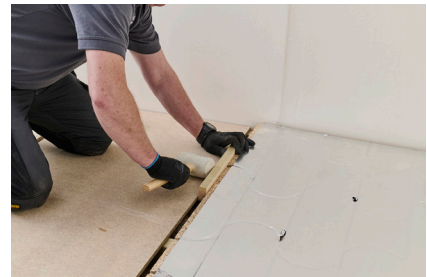
17. Replace the board and ensure the tongue and groove joints are fully closed, use a scrap block of timber and a mallet to tap the board to assist if required, take care not to damage the tongue or groove.
