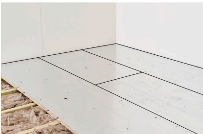
20. When starting each of the subsequent rows it is important to ensure that the board end joints are staggered as shown, preferably as a half-lap brick bond pattern.
