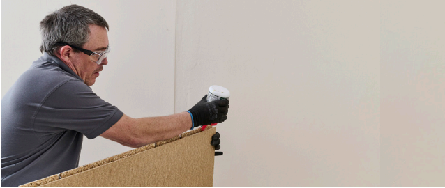
15. Apply PU adhesive to the tongue and groove joint only when the boards will join. Be careful not to apply the glue too close to the pipe channels, overspills will need to be cleaned out prior to installing the pipe.
