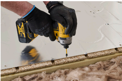
18. Fix the board down as previously done and remember to leave a 10mm gap at the wall edges.
