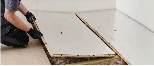
14. Place the board to check correct size and alignment, paying close attention the alignment of the channels.
