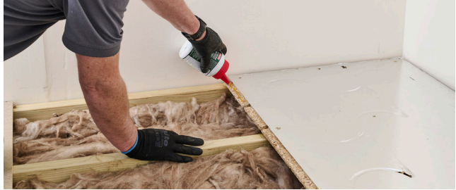
15. Apply PU adhesive to the tongue and groove joint only when the boards will join. Be careful not to apply the glue too close to the pipe channels, overspills will need to be cleaned out prior to installing the pipe.
