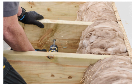
22. At the point where the flow and return pipework penetrates the floor an access point will need to be left, either in the room or just outside in the adjacent room or via the floor below. This is to facilitate the installation of the flow and return pipe-work through the floor void.
