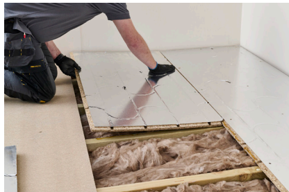
17. Replace the board and ensure the tongue and groove joints are fully closed, use a scrap block of timber and a mallet to tap the board to assist if required, take care not to damage the tongue or groove.
