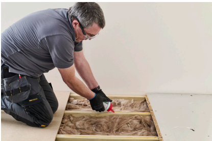
16. Apply PU adhesive to the top of each joist, where the board will be laid.
